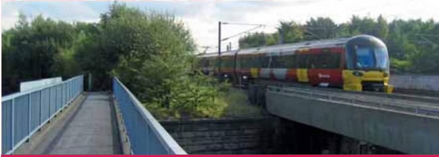
Footway and Railway at Armley Gyratory
