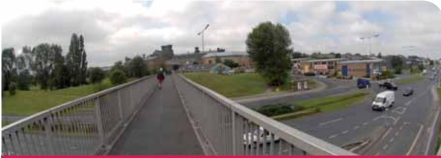
Footbridge across Armley Road / Canal Street
